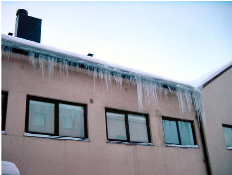
Figure 1. Building with icicles in Narvik. No pedestrian area below.
